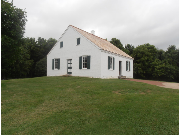
The Dunker Church today at Antietam National Battlefield
